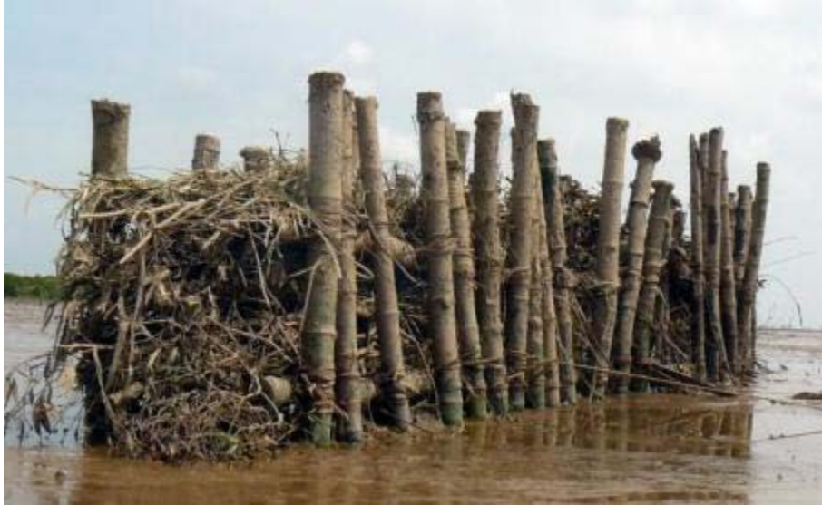
Figure 4: Cross section and seaward side of the bamboo fence
