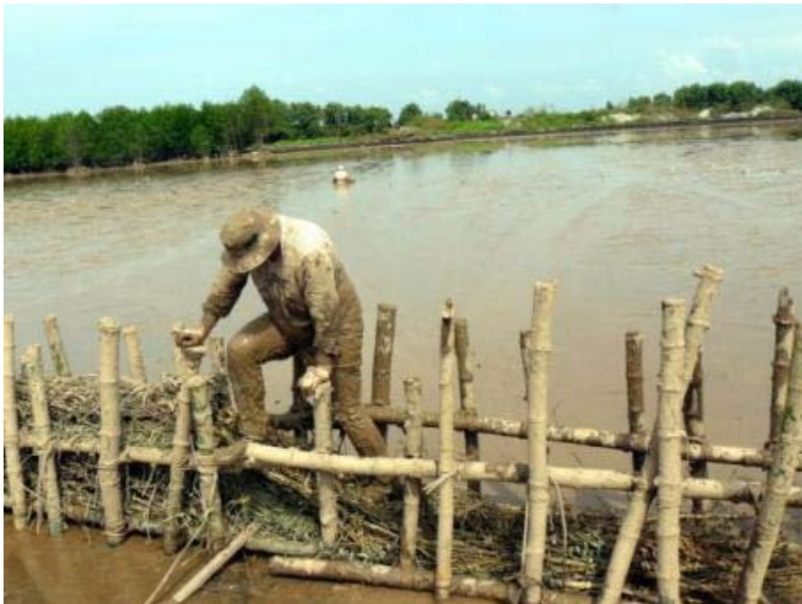
Figure 30: Installation and compacting of the bundles
