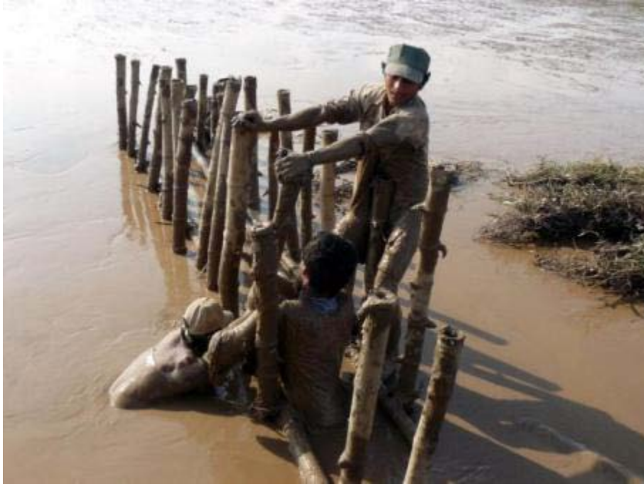
Figure 25: Fixing of the horizontal bamboo poles
