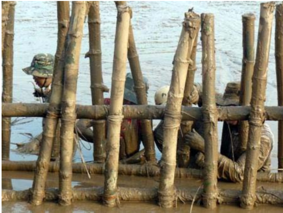
Figure 27: Preparation of the connections
