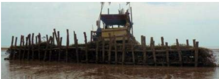
Figure 3: Front view; landward side of the bamboo fence
