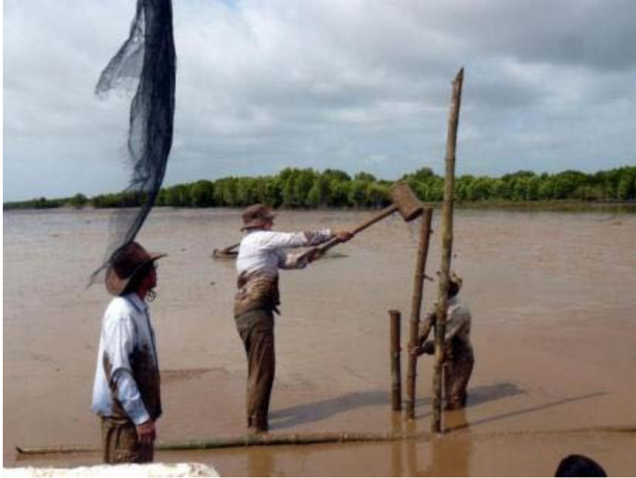
Figure 14: Installation using a sledge hammer
