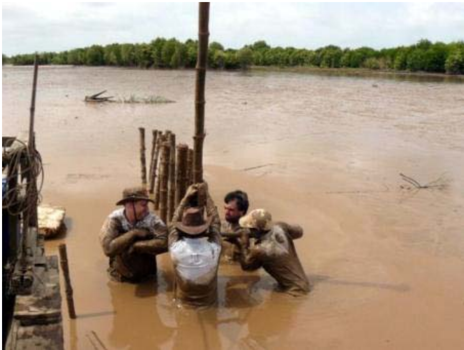
Figure 21: Installation using pressing technique with horizontal bar
