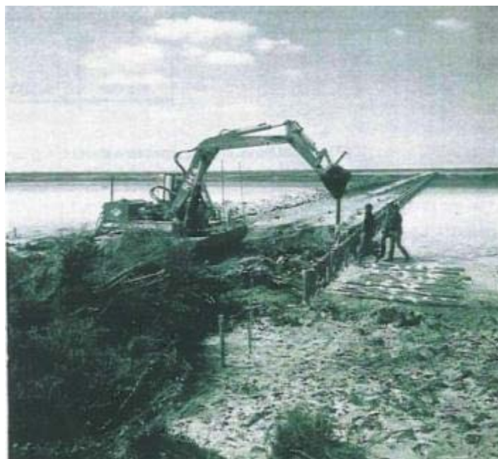
Figure 39: Installation of vertical poles using a dredger bucket
