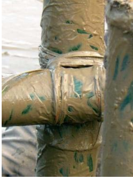
Figure 8: Joint made with rattan stripes
