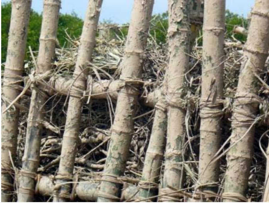
Figure 6: Side view of the bamboo fence
