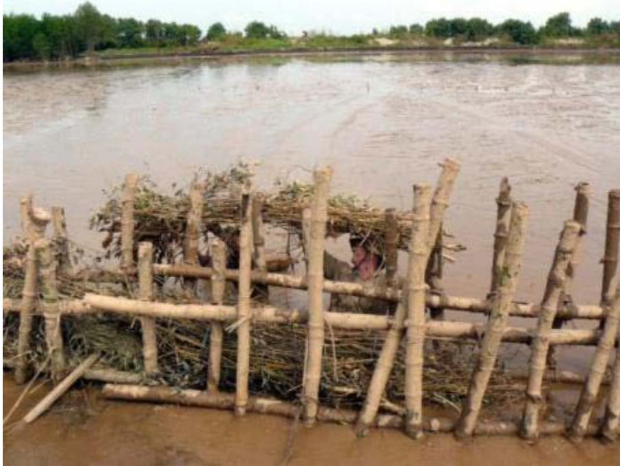
Figure 29: Installation of the bundles
