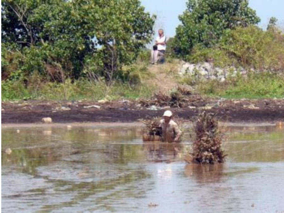
Figure 11: Material transport (bundles) to the construction site
