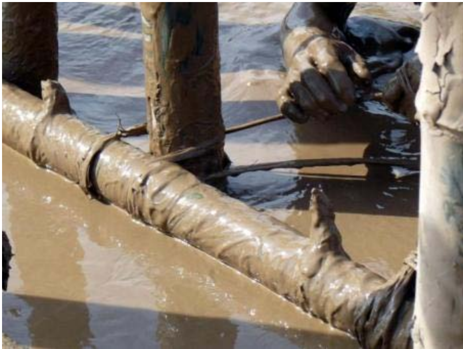
Figure 7: Connection of the horizontal bar to the vertical poles
