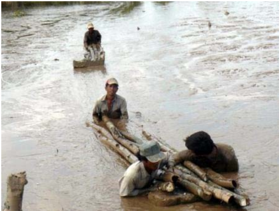
Figure 10: Material transport (bamboo) to the construction site
