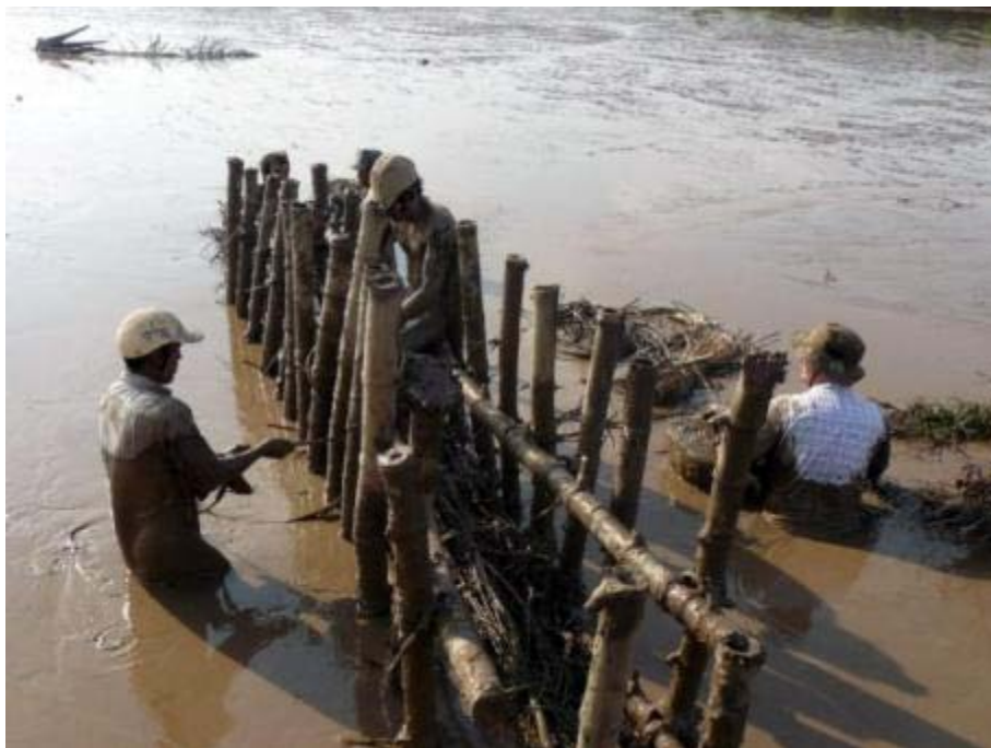
Figure 28: Preparation of the connections of the upper horizontal pole
