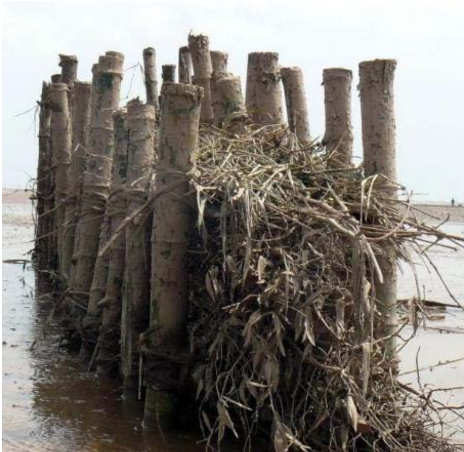
Figure 5: Cross section of the bamboo fence
