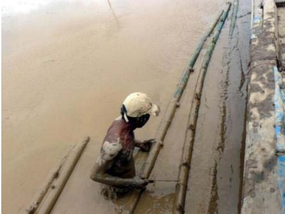
Figure 13: Cutting of excess material from the bamboo nodes
