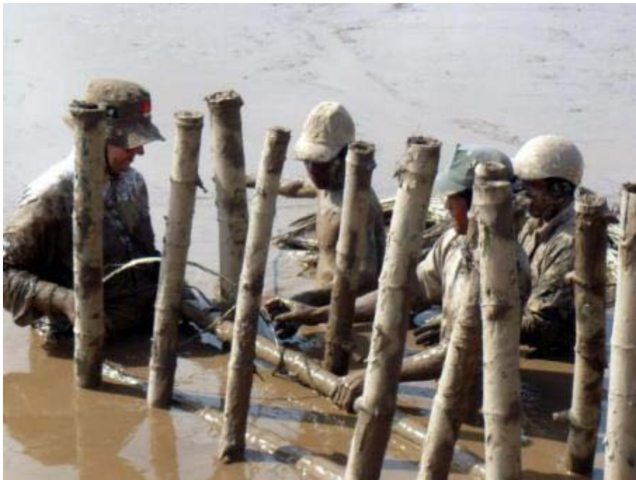
Figure 26: Connection of the horizontal bamboo pole
