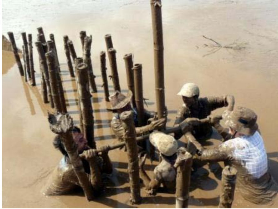
Figure 22: Installation of the second row
