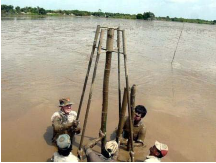
Figure 16: Installation using the head ram with four people
