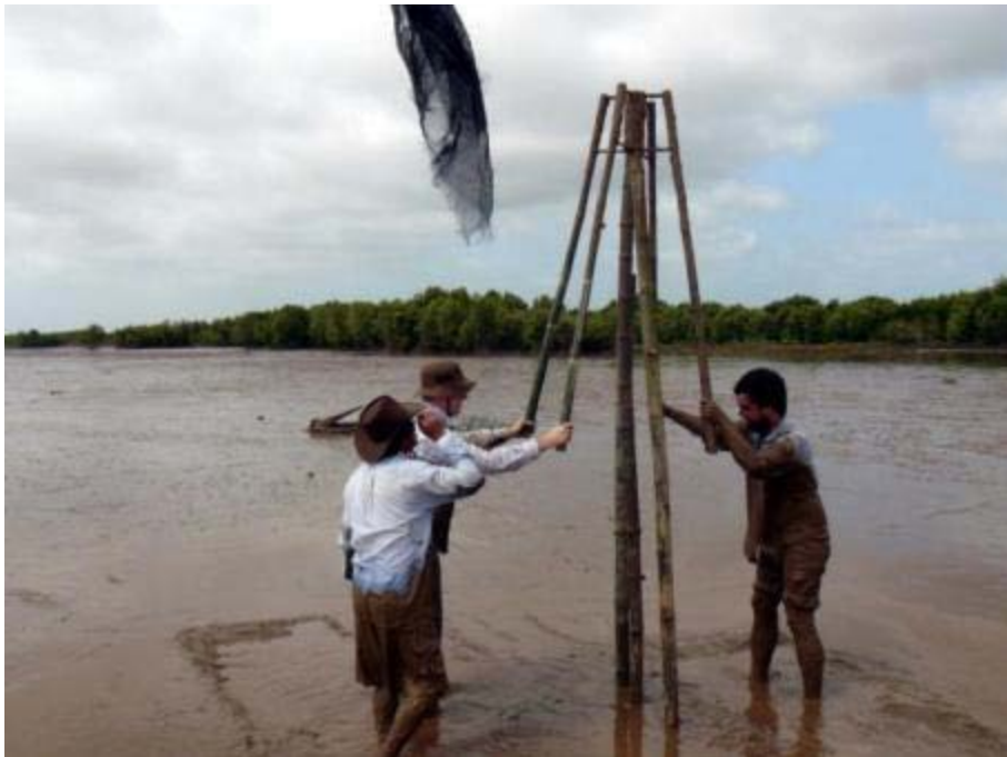
Figure 15: Installation using the head ram with two people
