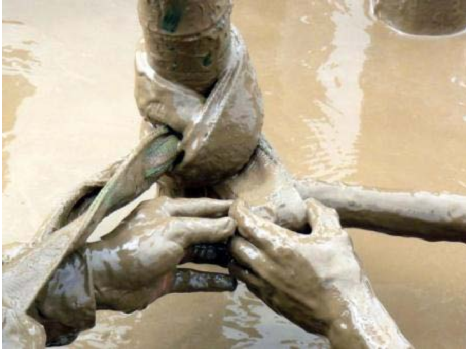
Figure 20: Fixing of the horizontal bar
