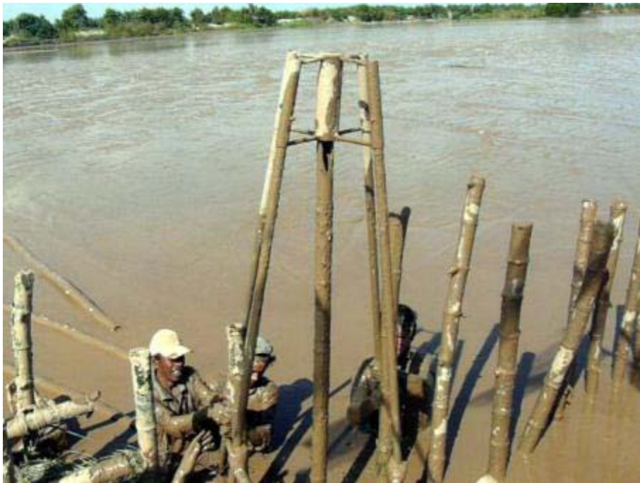
Figure 17: Installation of the second row using the head ram
