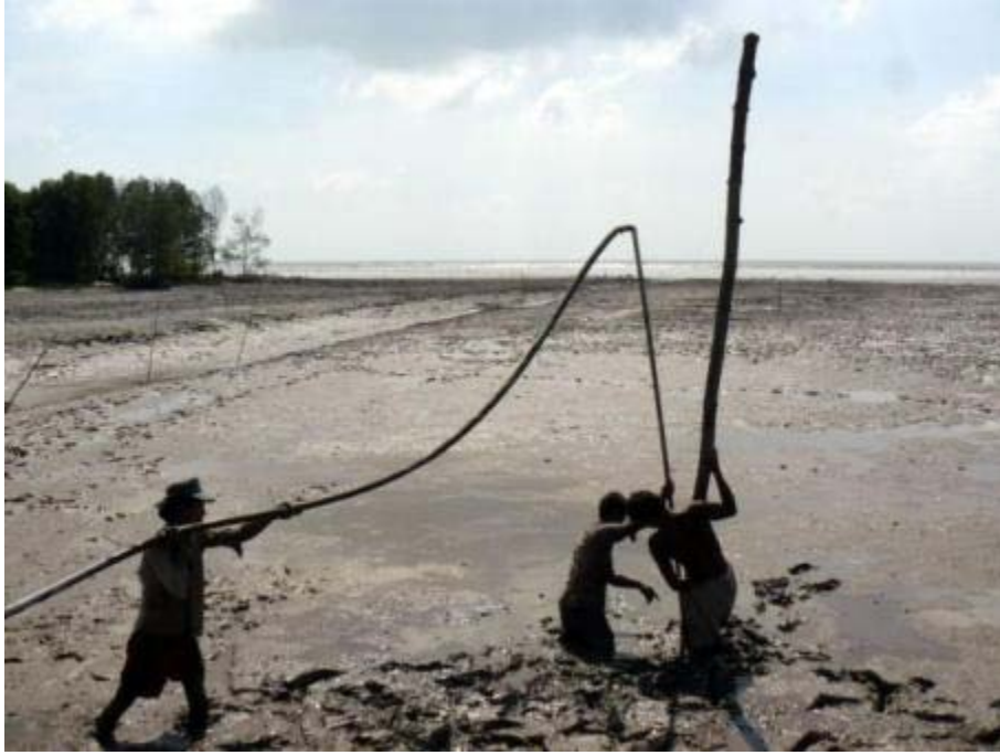
Figure 24: Installation using water pressure
