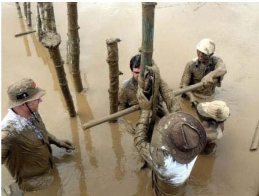
Figure 19: Installation using pressing technique with horizontal bar
