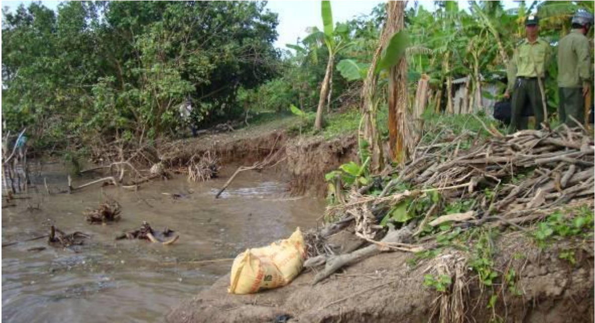
Photo B. Recent sea dike erosion at Khanh Hoi in U Minh District on the west coast of Ca Mau. This was previously protected by a seaward mangrove belt which disappeared rapidly over a period of several months (see Photo C below). The reason why the mangrove belt was breached here, but remains intact elsewhere is unknown.
