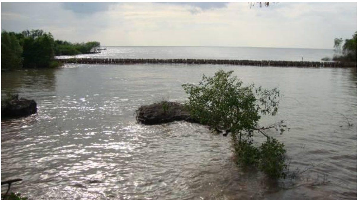
Photo B. Recent sea dike erosion at Khanh Hoi in U Minh District on the west coast of Ca Mau. This was previously protected by a seaward mangrove belt which disappeared rapidly over a period of several months (see Photo C below). The reason why the mangrove belt was breached here, but remains intact elsewhere is unknown.
