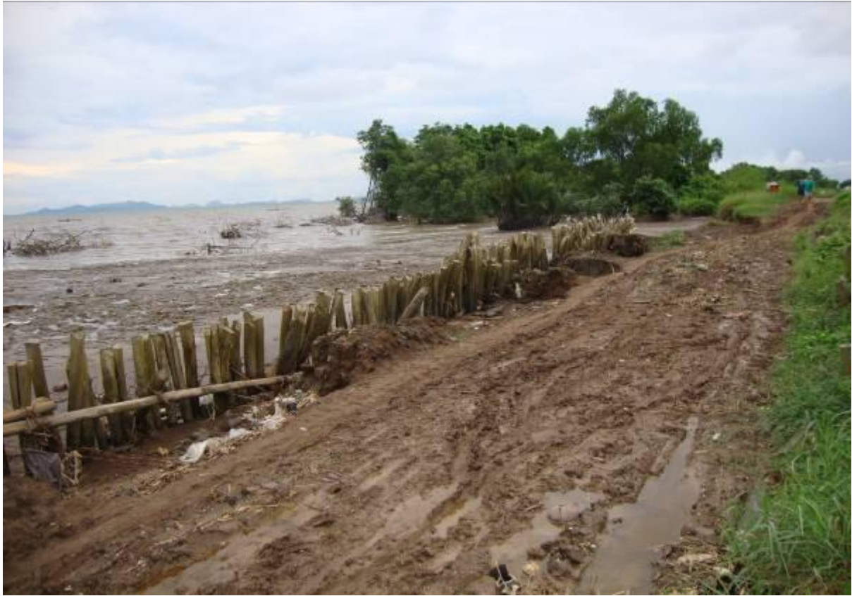
Photo A. An erosion site in Hon Dat district, Kien Giang province. The sea dike is exposed to the sea, with agricultural crops to the landward.
