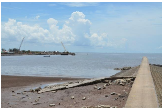
Figure 13: Existing sea wall at Ganh Hao which is currently (2014) being extended.
