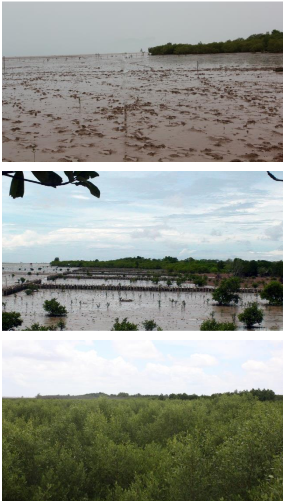
Figure 7: Erosion site in Vinh Trach Dong at which T-shaped bamboo breakwaters were installed and Avicennia seedlings planted. Top: before intervention. Center: 6 months after T-shaped bamboo breakwaters were installed. Bottom: 26 months after.
