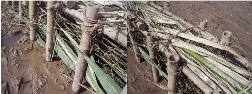
Figure 13: Nypa leaves as bottom layer (left) and top layer (right) of the bundles
