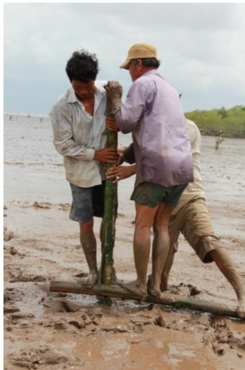
Figure 10: Installation of the vertical poles
