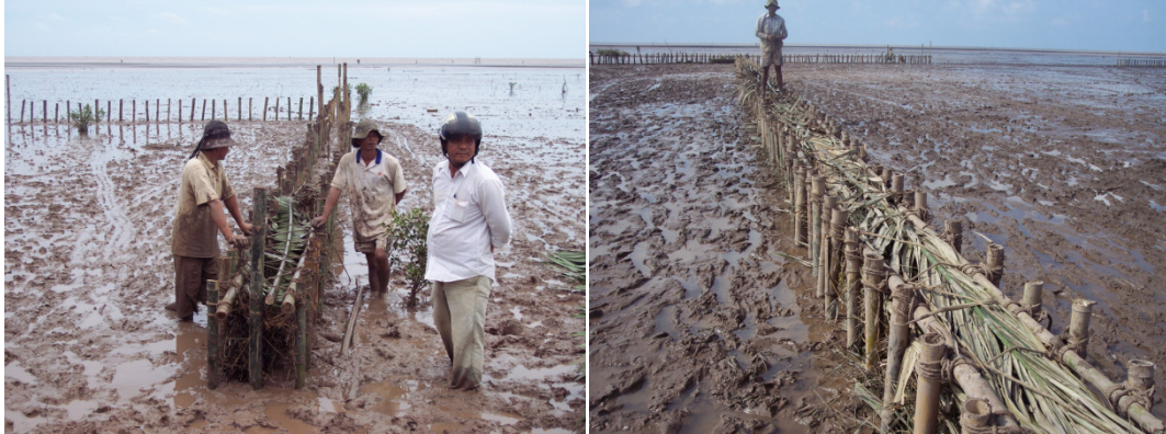
Figure 12: Different grades of completion of the fences
