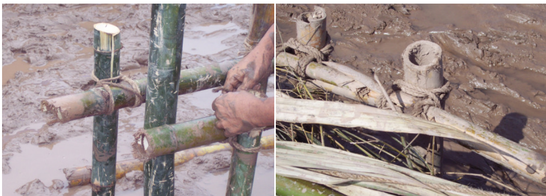
Figure 14: Joint lashes with jute rope
