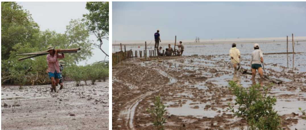
Figure 8: Transport of the bamboo and the bundles through the mud
