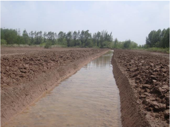
June 2011: The early stages of canal dredging.
