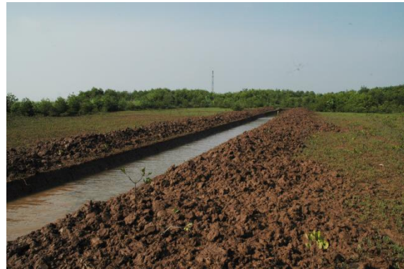
June 2011: The early stages of canal dredging.
