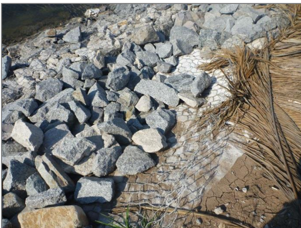
Figure 3-13 Rip-rap prevent and geotextile, sluice new 1 (Sikora) Figure 3-14 Paving stones and scour hole, sluice 8 (Sikora)
