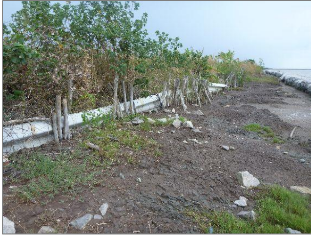
Figure 3-6 First aid measures of dike toe protection and gabions km (-16) (Sikora)
