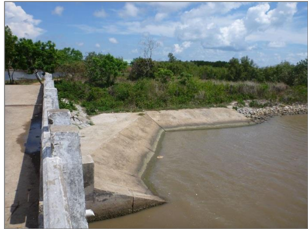
Figure 3-16 Overview of typical revetment arrangement, sluice 7 (Sikora)
