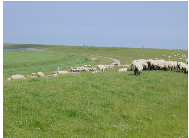
Fig. 1: Modern Seadike in Germany (photo: Schüttrumpf)
