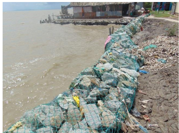
Figure 1a and 1b: Mangrove plantation and gabions shore protection in Kien Giang (Source: Province of Kien Giang)
