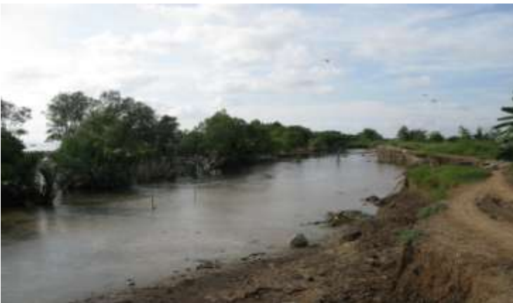
Photo 18: Excavation trench along the dyke
