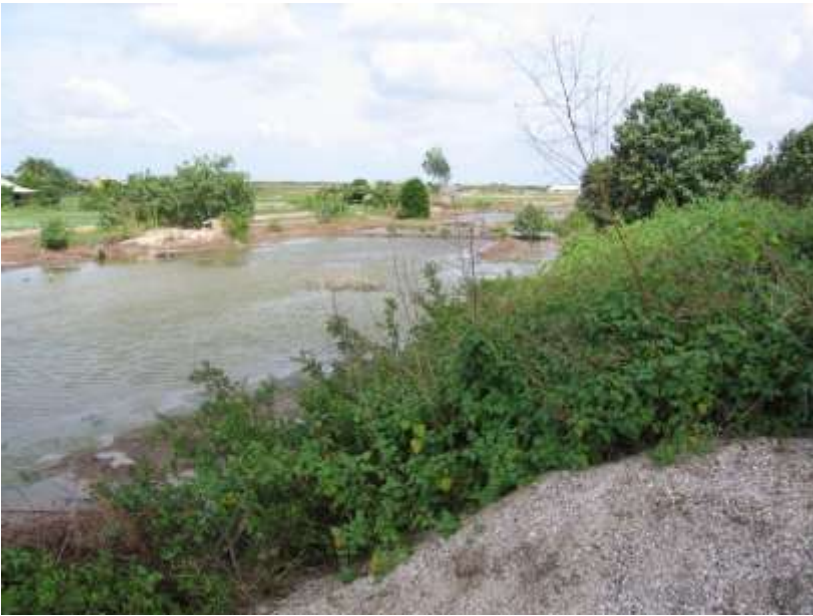
Photo 8: Landside slope of dyke
