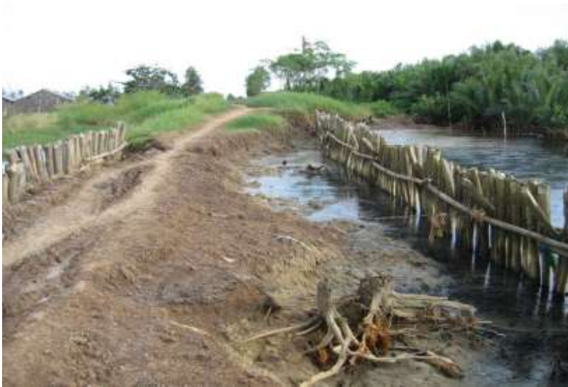
Photo 14: Collapsed dyke
