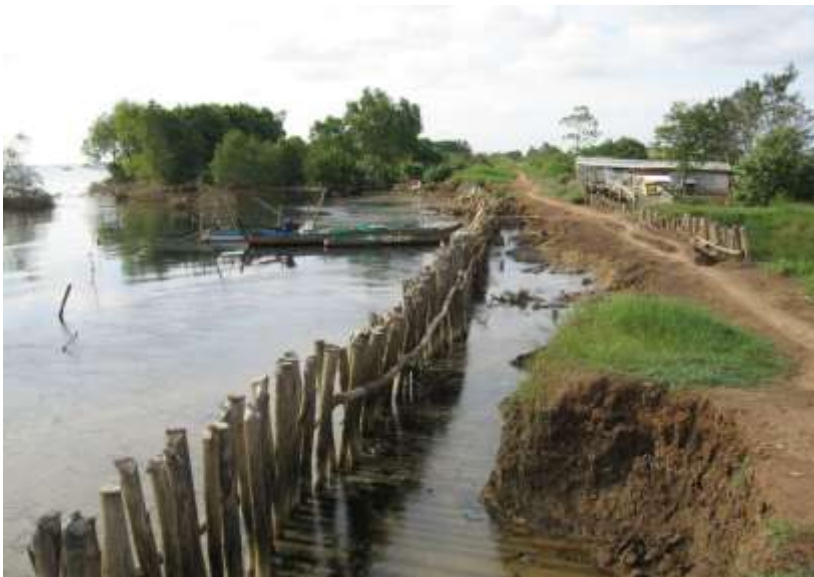
Photo 15: Eroded dyke
