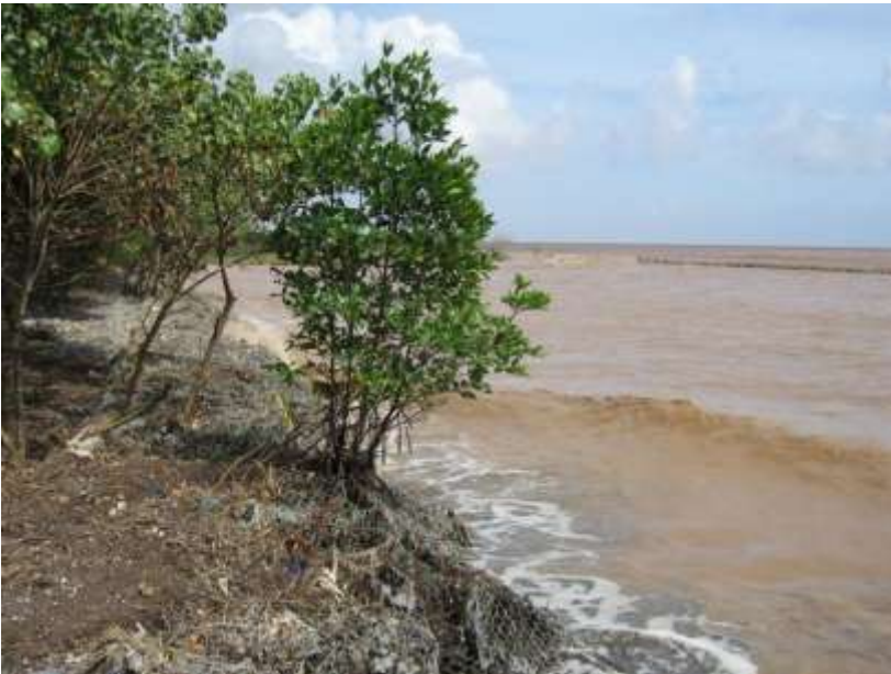
Photo 5: Eroded Foreshore, Protection with gabion mattresses
