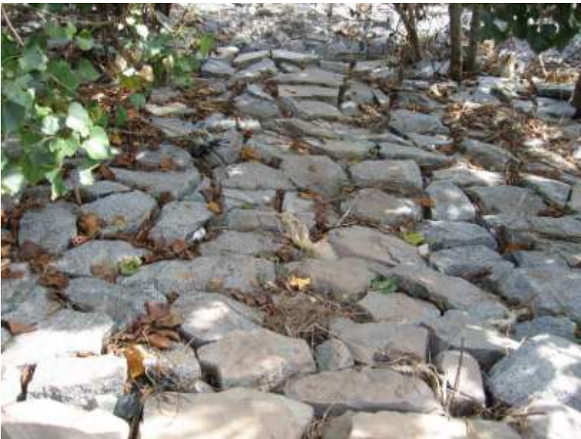
Photo 7: Slope protection with rip-rap
