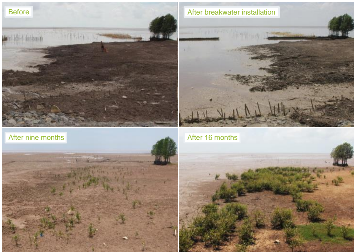
Figure 7: Restoration of eroded floodplain through bamboo breakwaters (from top left to bottom right): before, after installation of breakwaters, first natural regeneration after nine months, and after 16 months. (Photos: R. Sorgenfrei ©GIZ)
