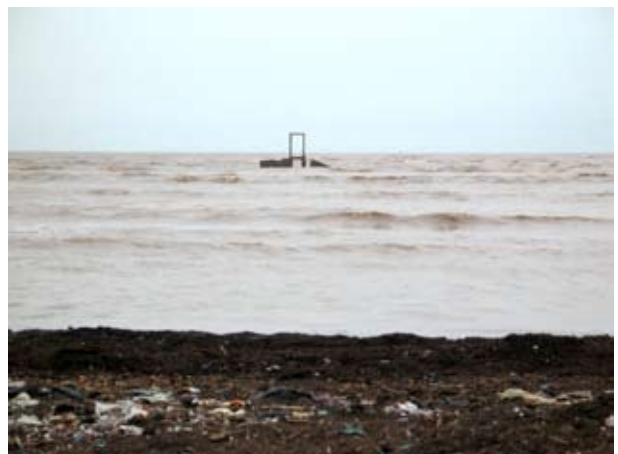
Figure 5: The sluice gate, which was at the dyke 10 years ago, is now 300 m from the coastline.
