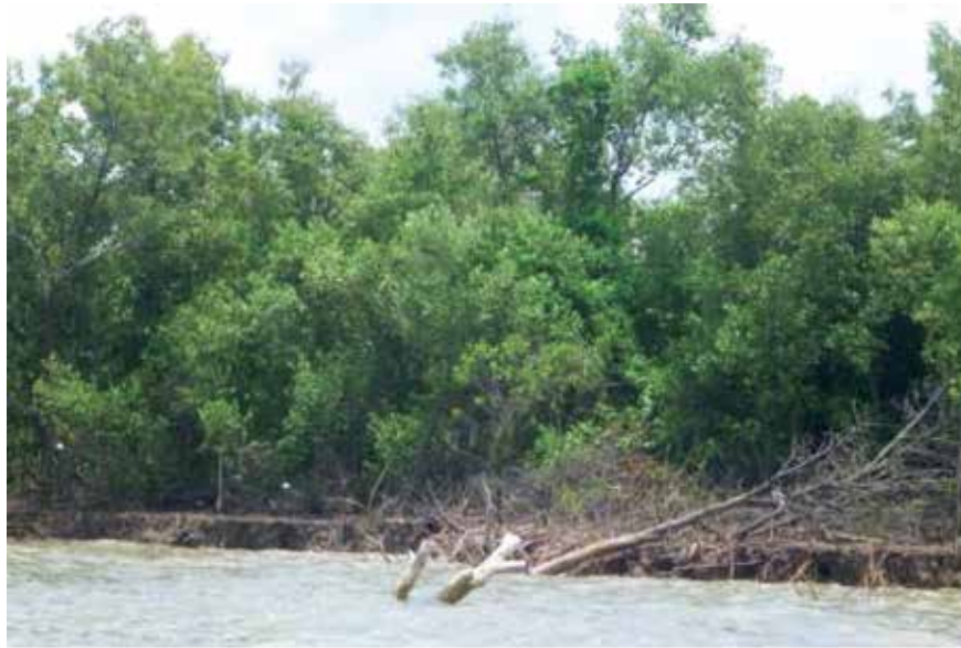
Severe Erosion; showing very gently sloping landward edge with steeply sloping seaward margin, an erosion scarp >1 metre in height, no mangroves present in front of the scarp, exposed sediment layers, exposed roots of mangroves, fallen trees.
