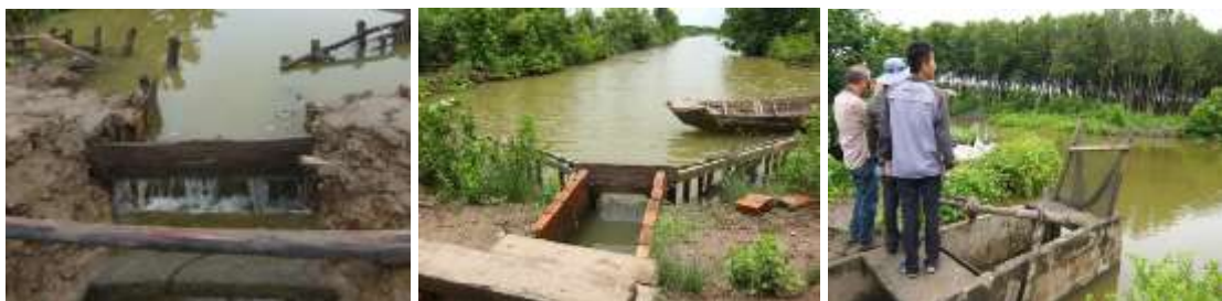
Figure 8. Sluice gates at extensive ponds in southern districts. The sluice gate design influences tidal water exchange rate and, if they leak, pond depth as the tide subsides. The size, location and number also effect water circulation and mixing patterns.
