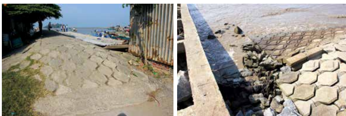
Figure 27: Ends of the dike construction near Hon Da Bac island
