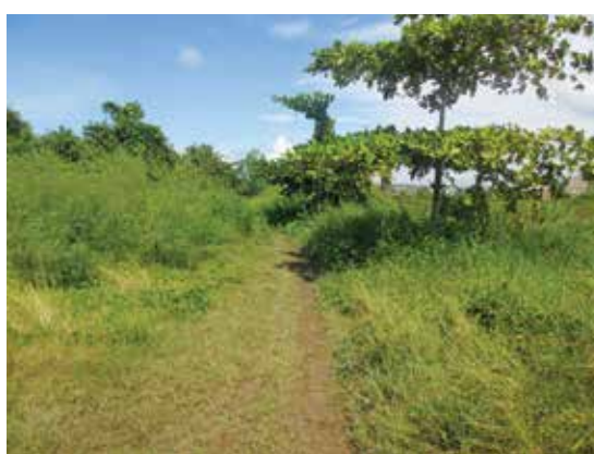
Figure 7: View along the dike
