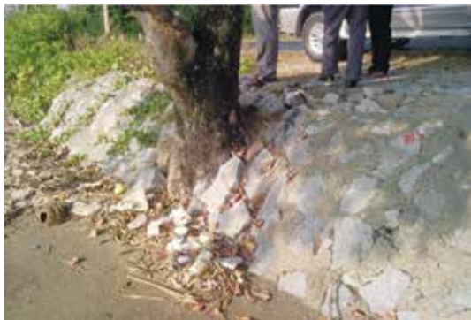
Figure 3: Highly damaged dike revetment (left) and dike revetment with concrete slabs (right) [Heiland & Schüttrumpf, 2009]
