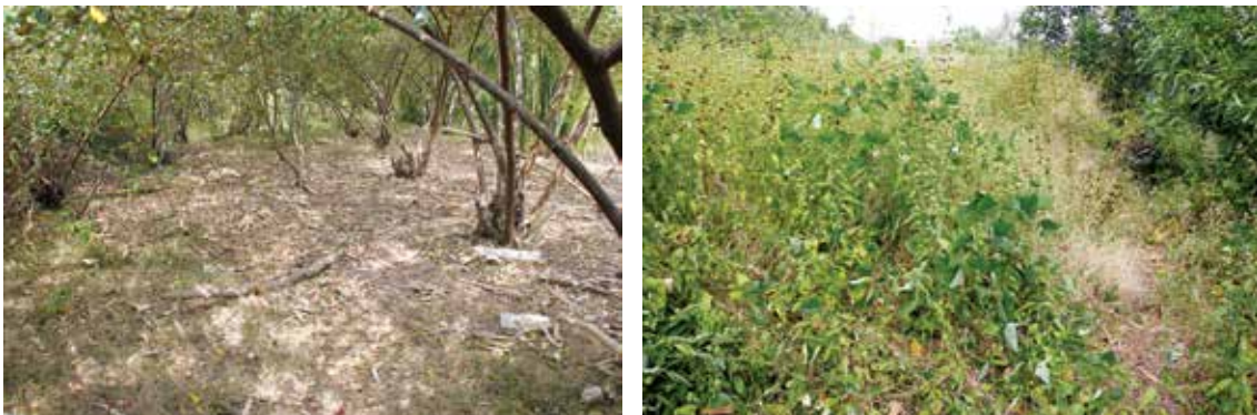
Figure 28: View along the dike line (06.01.2014 #9 left and #7 right)
