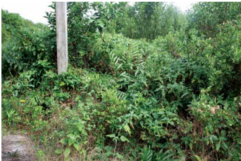
Figure 12: View along the dike line (03.01.2014 #2)
