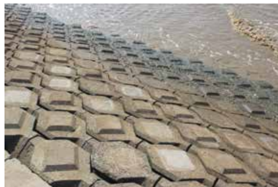
Figure 25: Concrete slab revetment on dike crest and seaward slope (left) and missing roughness elements on the seaward slope (right)
