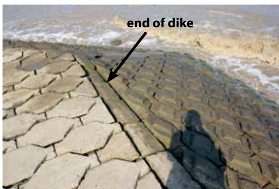
Figure 25: Concrete slab revetment on dike crest and seaward slope (left) and missing roughness elements on the seaward slope (right)
