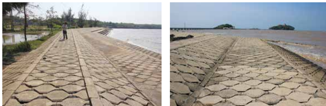
Figure 23: View along the dike line (20.01.2014 #2 left and #4 right)
