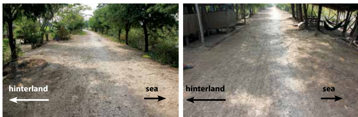
Figure 19: View along the dike line (06.01.2014 #1 left and #5 right)
