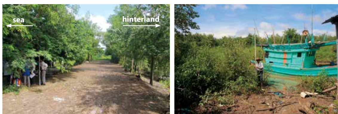
Figure 6: View along the dike (left) and dike foreland (right)
