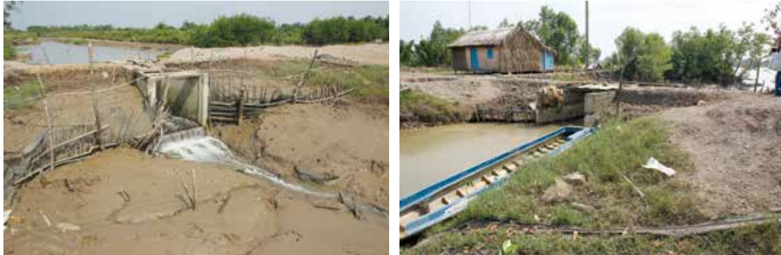
Figure 16: Sluice gate photographed from front (left) and back (right) (03.01.2014 #9)
