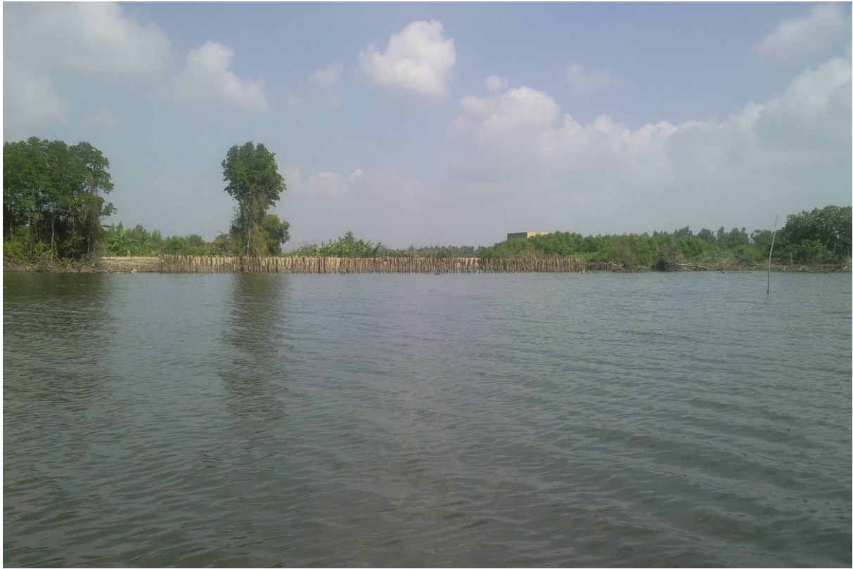
Fig.7: Protection of eroded area by wooden fences
