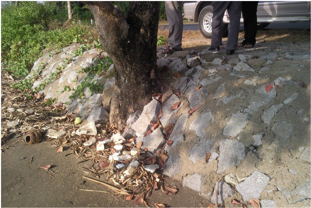
Fig.11: Coastal revetment south of Ha Tien Town
