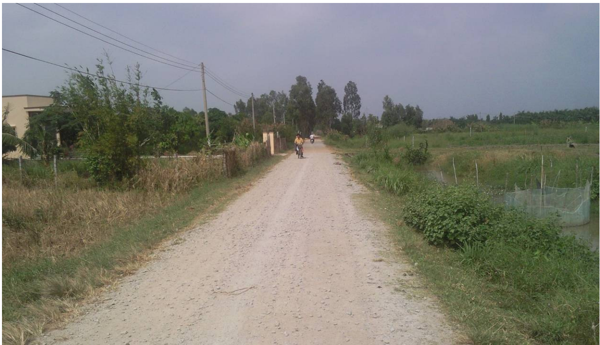
Fig.3: National defence dyke, Vinh Quang , Rach Gia City
