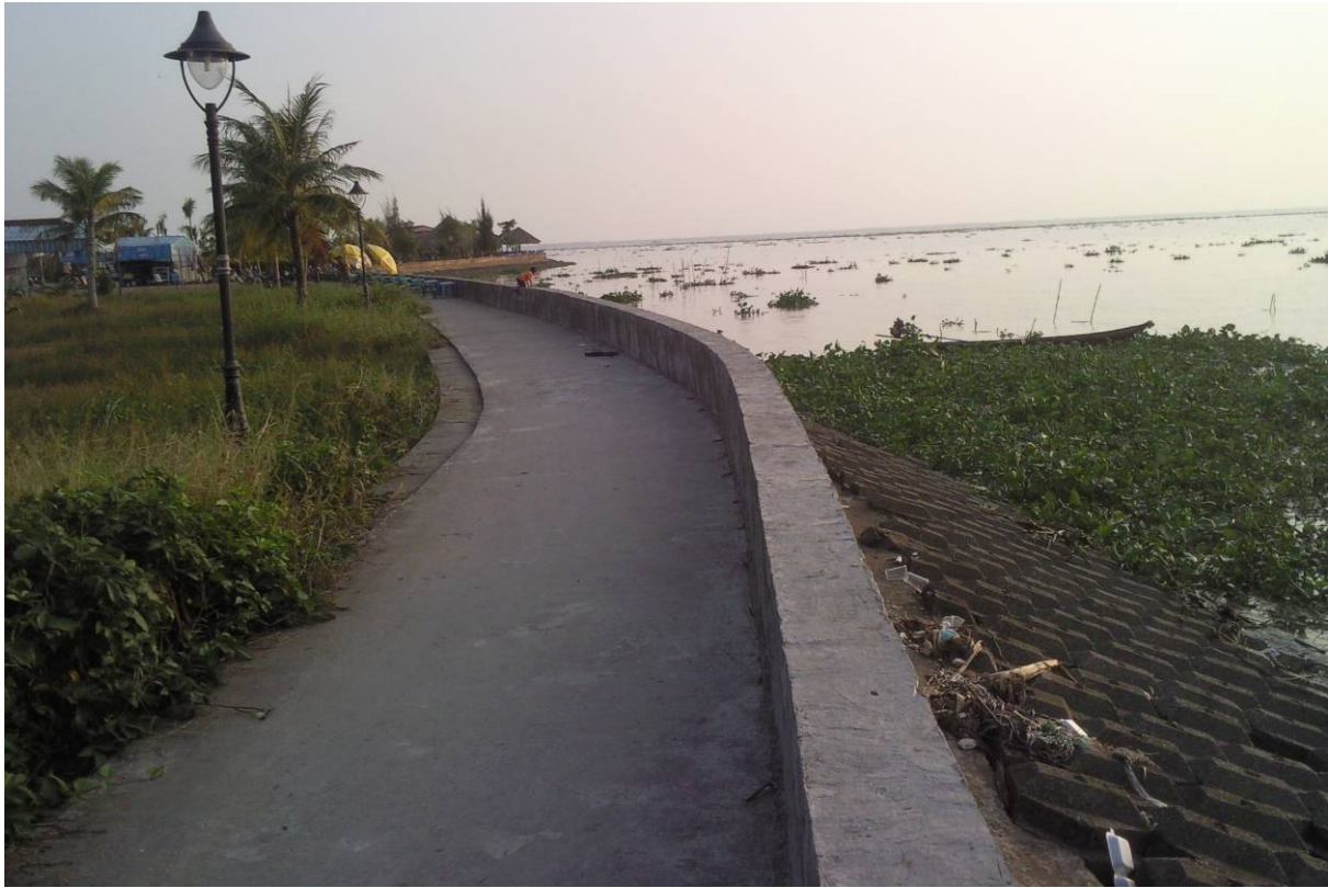
Fig.17: Seawall in Rach Gia City
