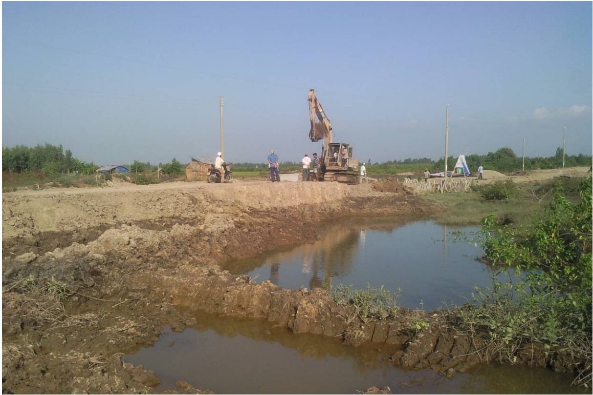
Fig.10: Dyke construction works close to T6 canal
