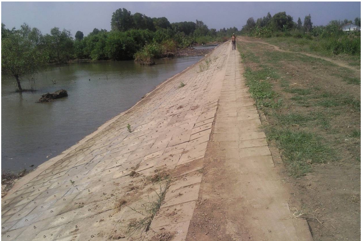
Fig.8: New coastal dyke in Hon Dat district
