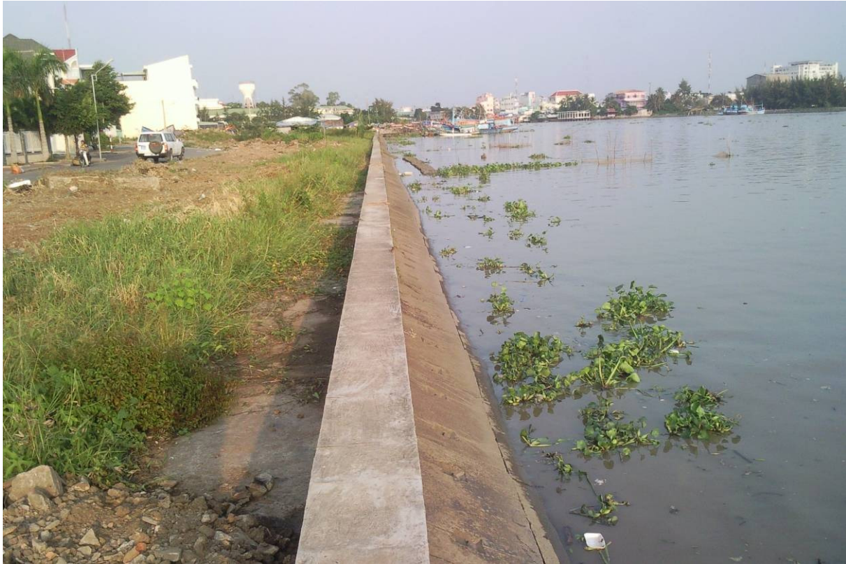
Fig.16: Seawall in Rach Gia City
