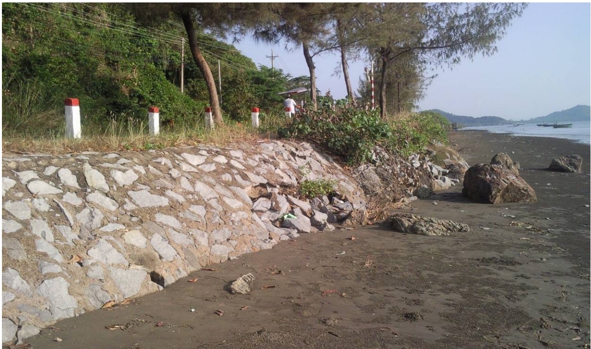
Fig.12: Coastal Revetment south of Ha Tien Town
