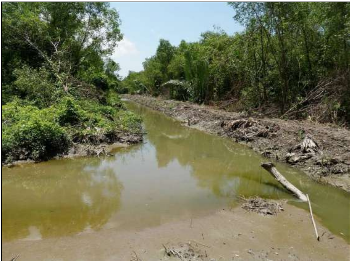
Figure 13: Unauthorised fish pond dug within a relatively wide and well developed mangrove, Vam Rang.
