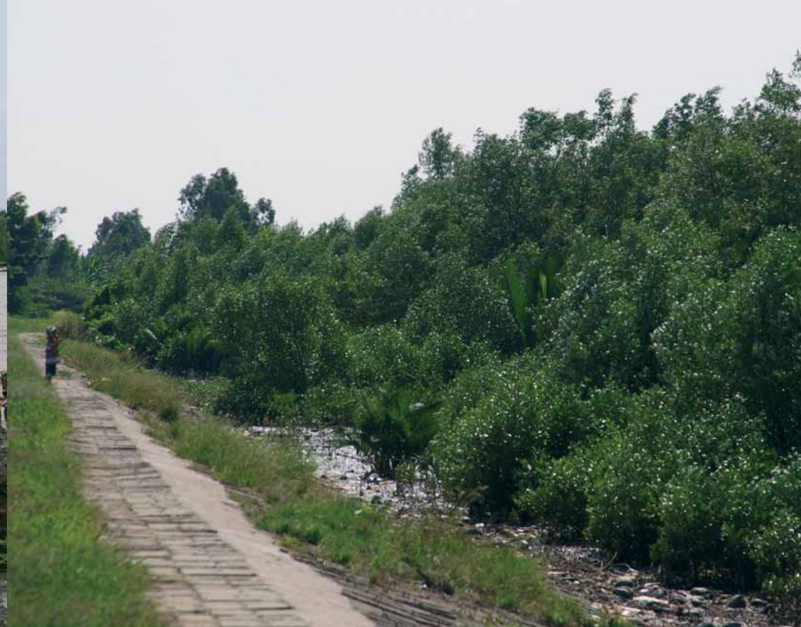
The coastal demonstration model after two years. A dyke and melaleuca protection fences were constructed and different species of mangroves planted.
