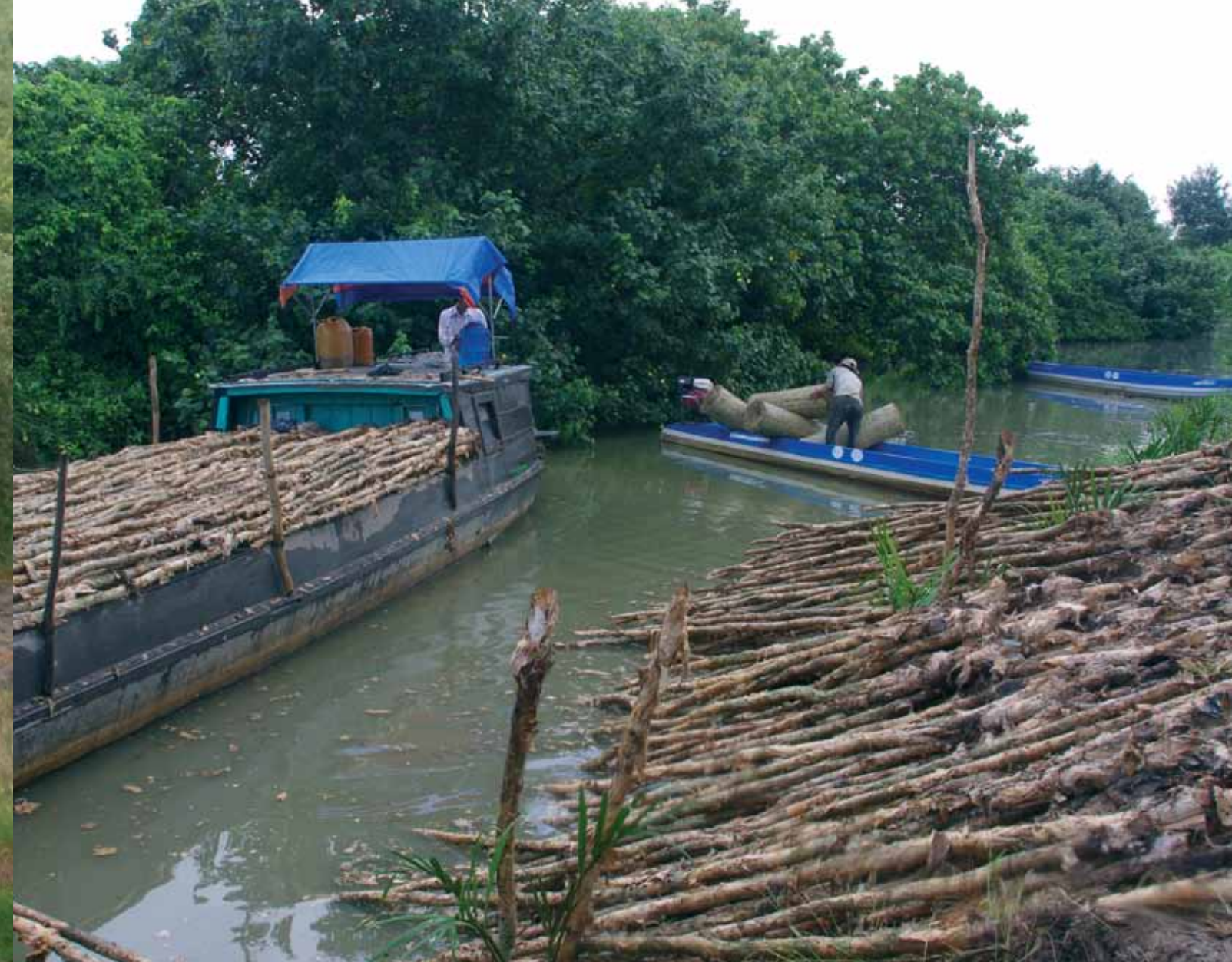
Boats transporting melaleuca poles and bamboo mats for the construction of mangrove protection fences.
