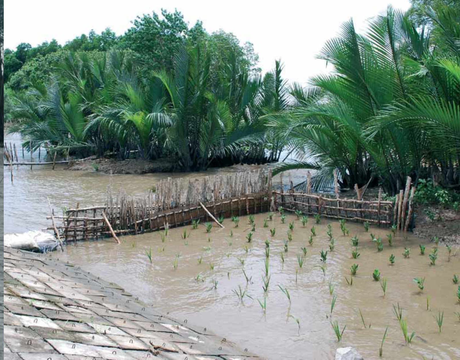
Sediment trap fences for areas of low erosion and for natural regeneration.
